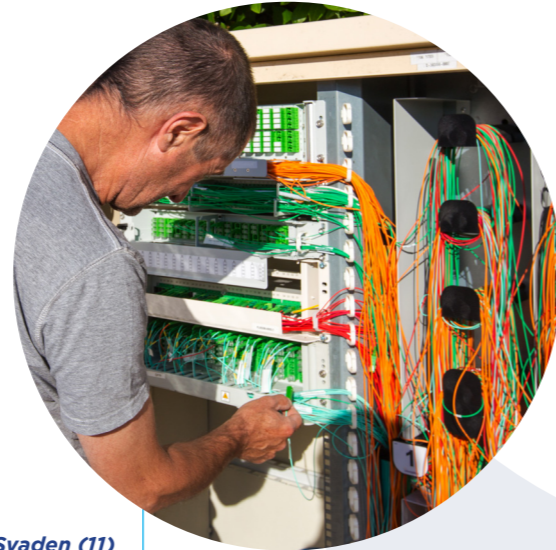
Syaden (11) Roll-out of fibre optic cables within the department
